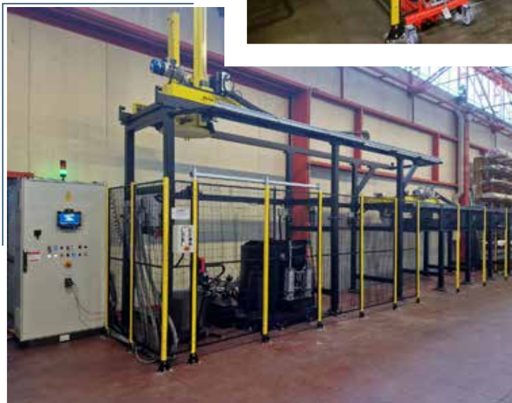
Plant with three discharge stations
